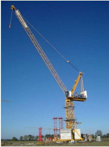
Tower cranes (including self erecting)
